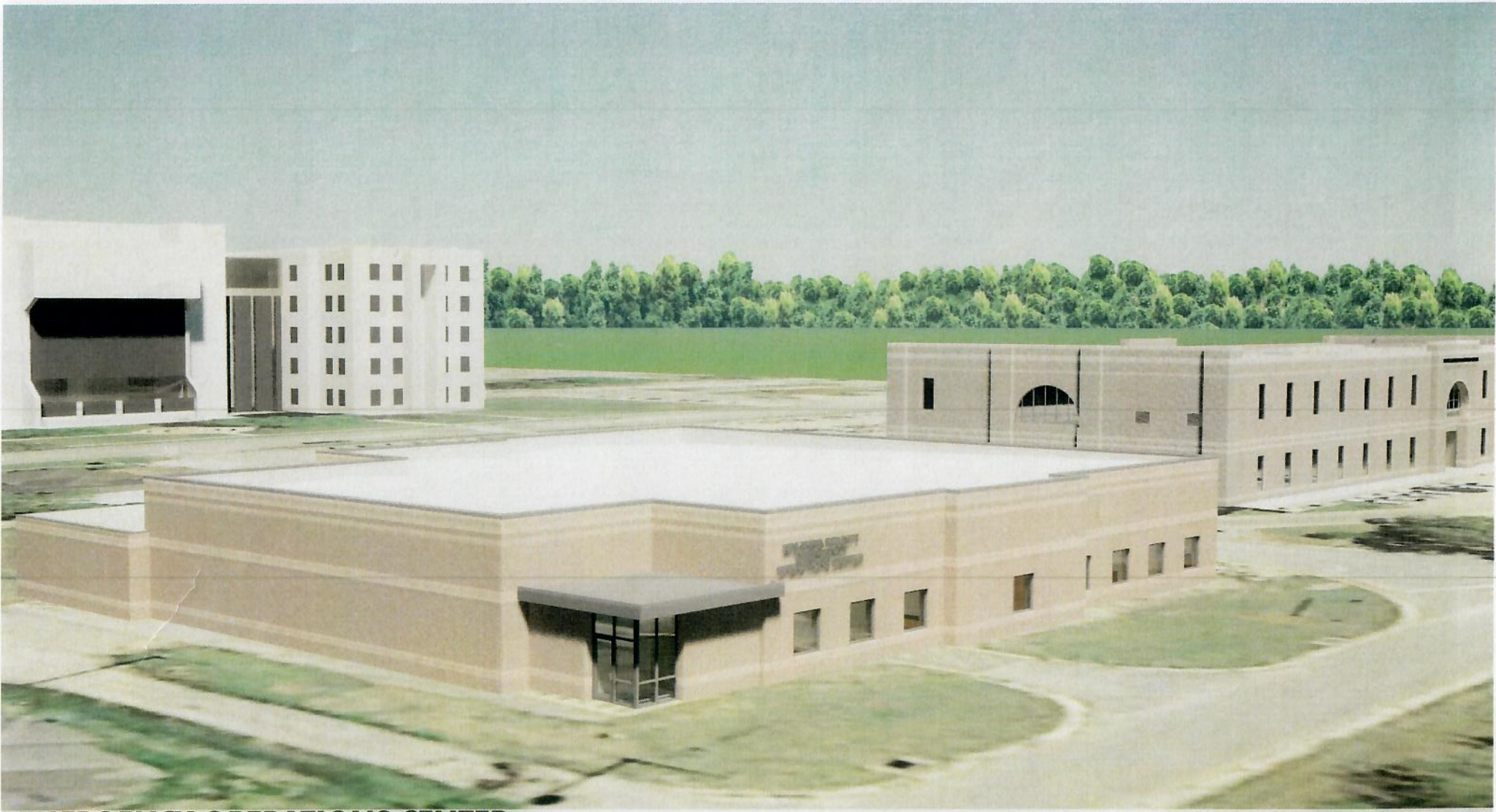
EMERGENCY OPERATIONS CENTER
